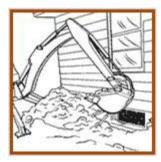
Mark a centerline on the foundation above the window. Dig the hole so it is centered across the window opening.
